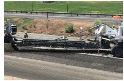
Hinging Swing Conveyor. 35' (10.66 m) Long 170 Degree Swing Arc
